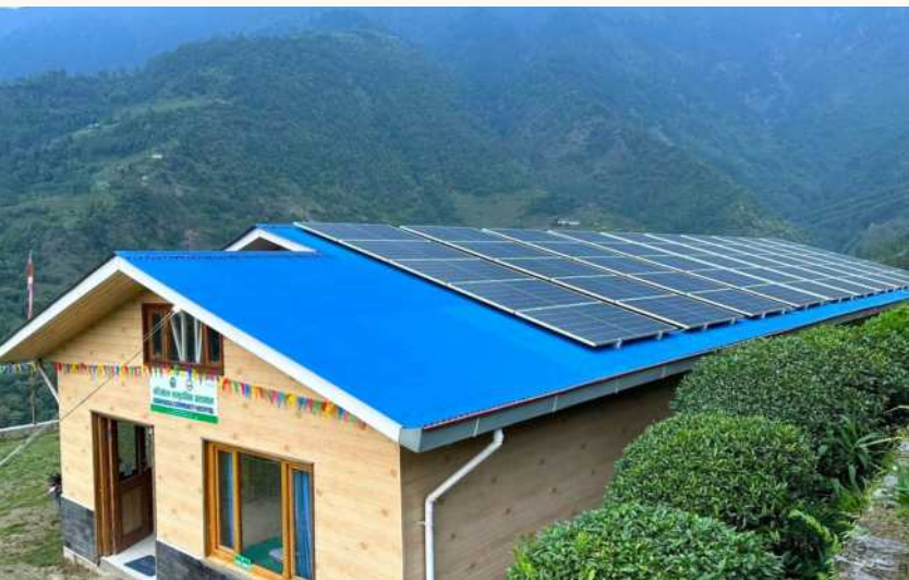
New Solar power
